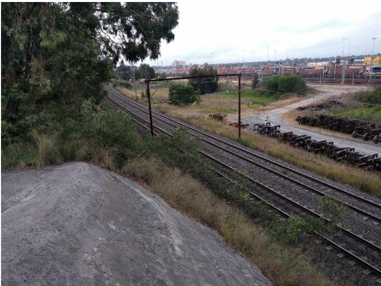
Photograph 10: Facing north from Mainline road over the Enfield rail yards, showing the possible swale area between rails where surface water may drain to.
