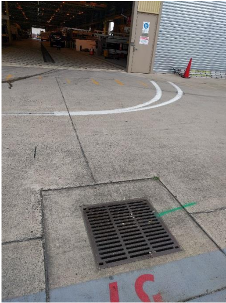
Photograph 5: Facing west, surface water drain (sample location SW03) at the eastern entrance to the main warehouse, showing the out going drainage channel from this location (green marking) to SW01.
